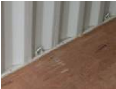
Container lashing points
